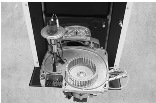
Abb. 34: Brenner in Serviceposition
